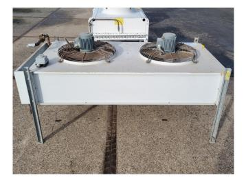
type LK HELPMAN 220-380-50 max. workingpressure 23 barg Groningen Holland electric defrost
